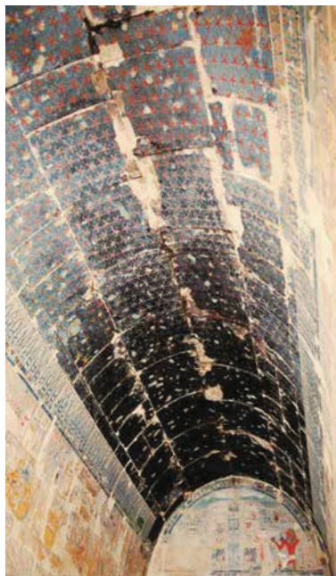
The corbelled vault hollowed out underneath to achieve a vaulted effect in the Barque Hall. The painted blue ceiling is covered with a layer of soot and, as the result of high temperatures, the yellow painted stars changed their color to red. These are remains of activity from the Byzantine times. (Far left and center) The Southern Chapel of the Great Theban Ennead, the Room of the Cult Statue and former Inner Sanctuary. In the Ptolemaic period, in this last room, all the original limestone blocks were removed and replaced with sandstone ones (Pawlicki, 2017).
